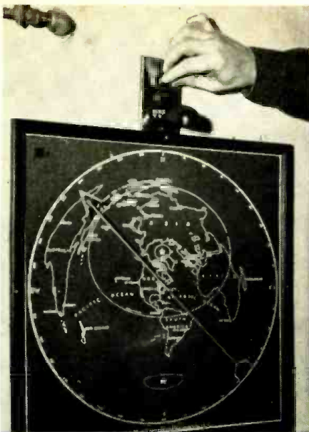
Fig. 6. The "on-off" switch, fuse, and pilot lamp are mounted at the beam-indicator map. The control switch is at the operator's desk. A selsyn drives the arrow.
